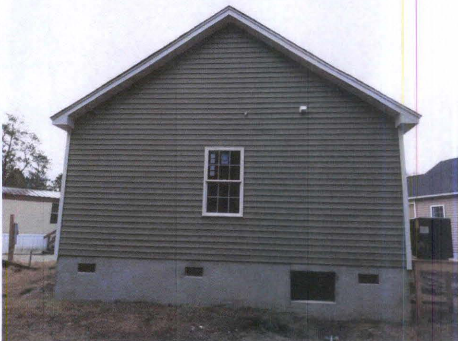
Photo Two Caption REAR VIEW
