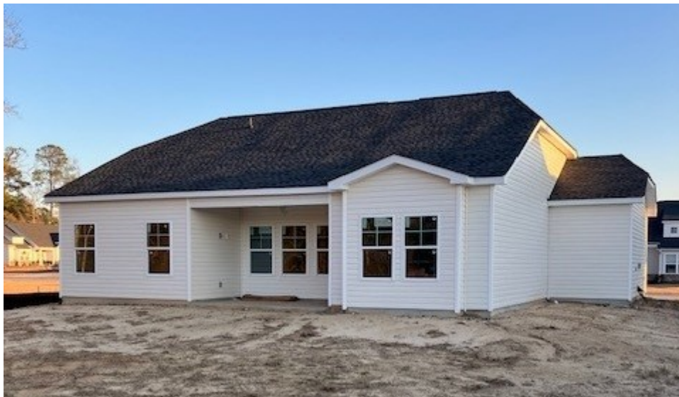
Photo Four Caption: REAR LEFT VIEW 01/04/2024
