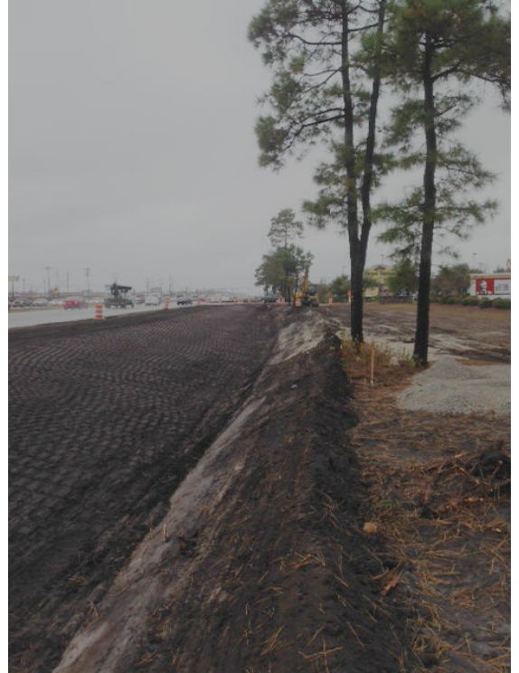
Hwy 501 undergoing a lane expansion project.
