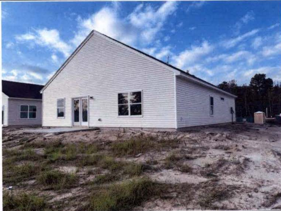
Photo Two Caption Rear View; 10-11-2022
