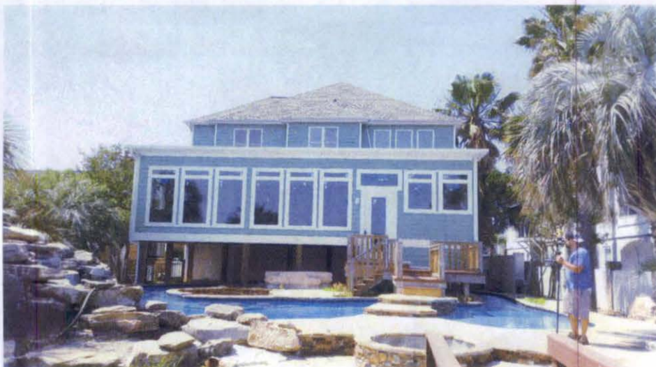
REAR VIEW (CREEK SIDE) PHOTO TAKEN 5/27/2016
