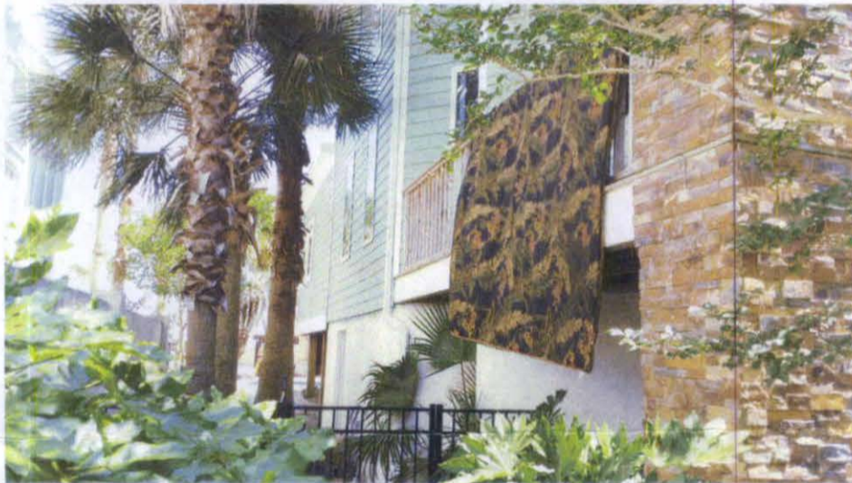
FRONT VIEW (STREET SIDE) PHOTO TAKEN 5/27/2016
