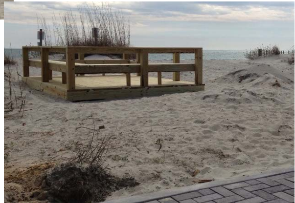
Redesigned seating areas have been installed.
