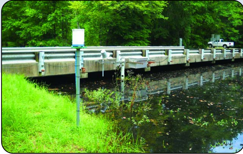
USGS Monitoring Station on Long Ave. Ext.
