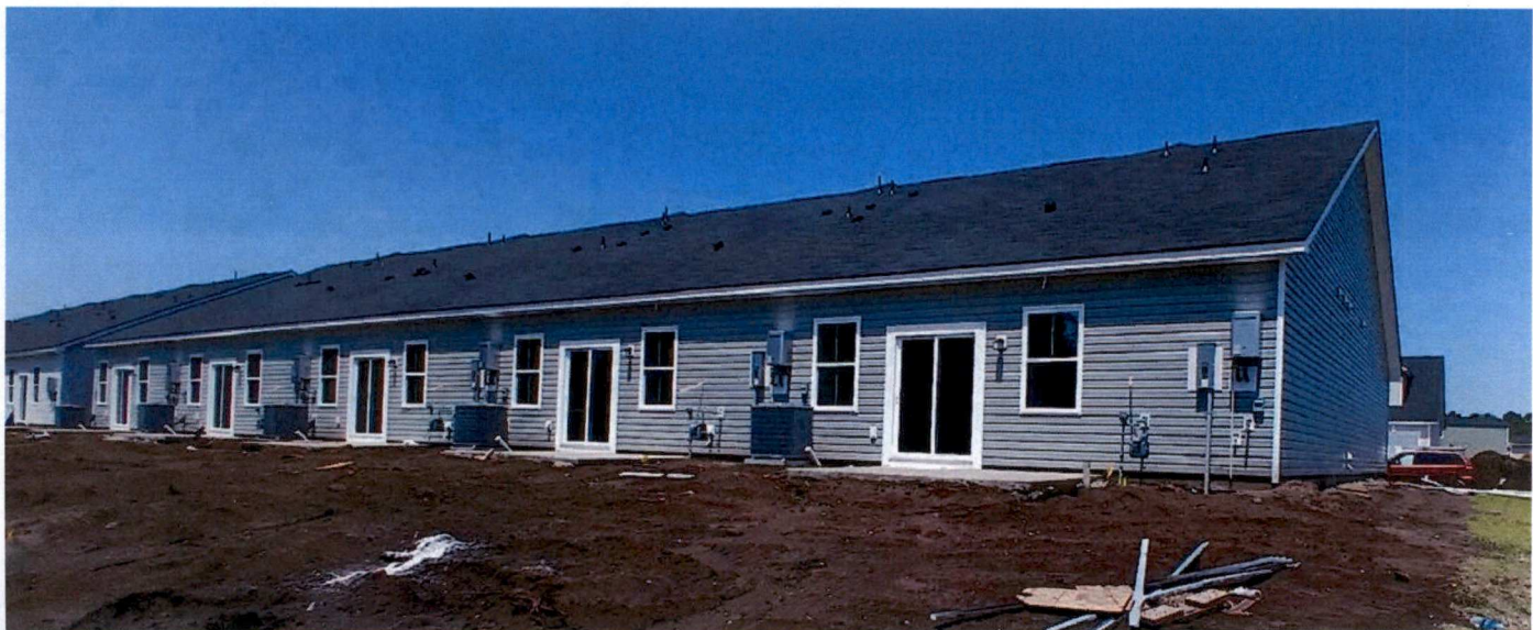
Photo Four Caption: REAR LEFT VIEW 05/07/2024
