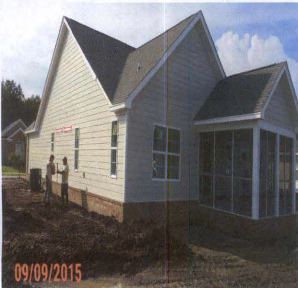
Right side HVAC Rear
