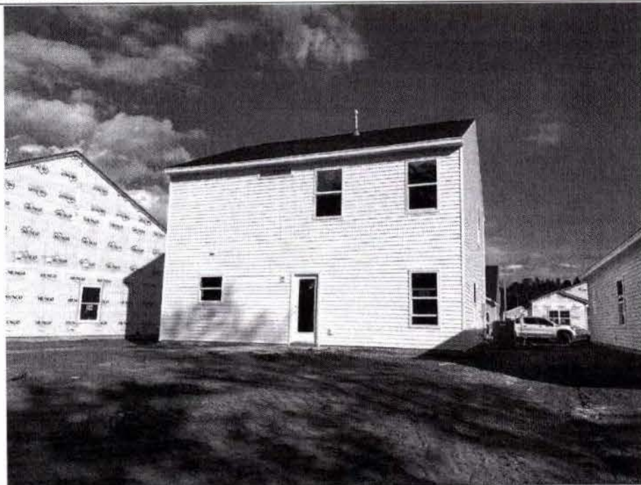
Photo Two Caption Rear View; 10-26-2022
