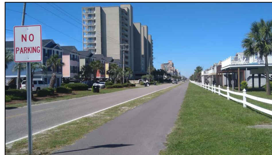
Waccamaw Drive Multipurpose Path - portion of the East Coast Greenway
