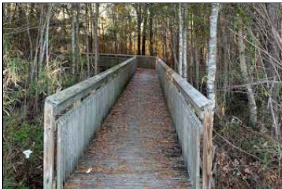
Example Boardwalk over wetlands in Horry County
