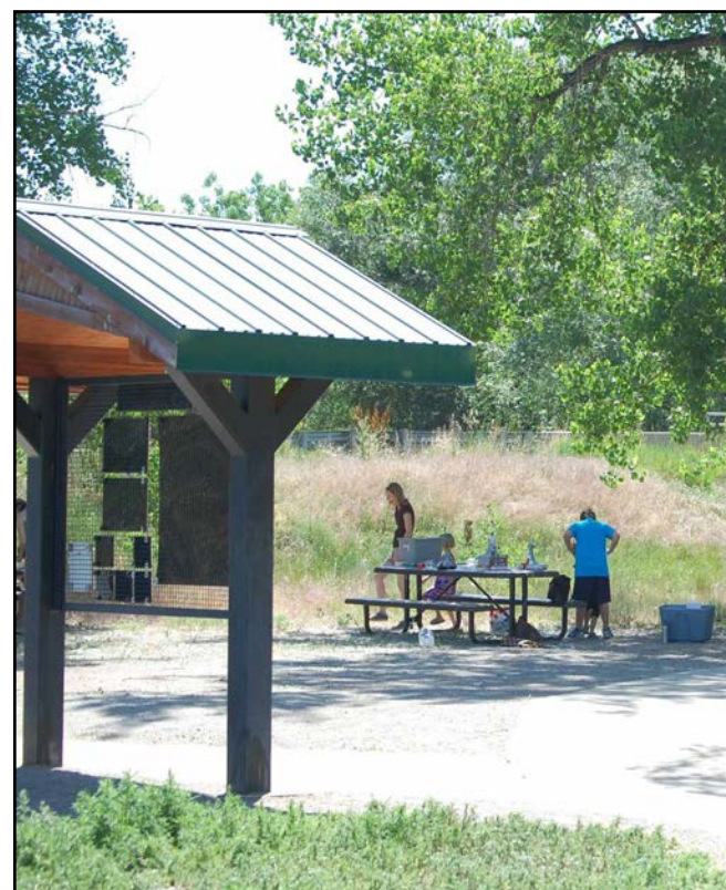
The Trailhead should allow for passive recreational uses and serve as a respite for trail users
