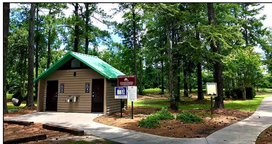
Restrooms and trailhead
