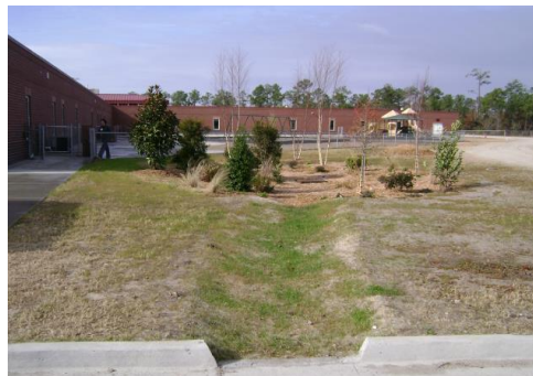
Bioretention Facility
