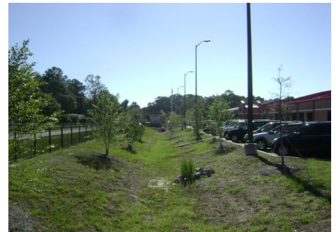
Infiltration Trench
