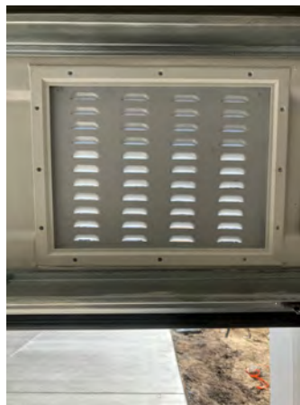
BACK OF NON-ENGINEERED FLOOD VENT
