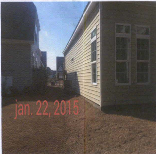
Right side HVAC
