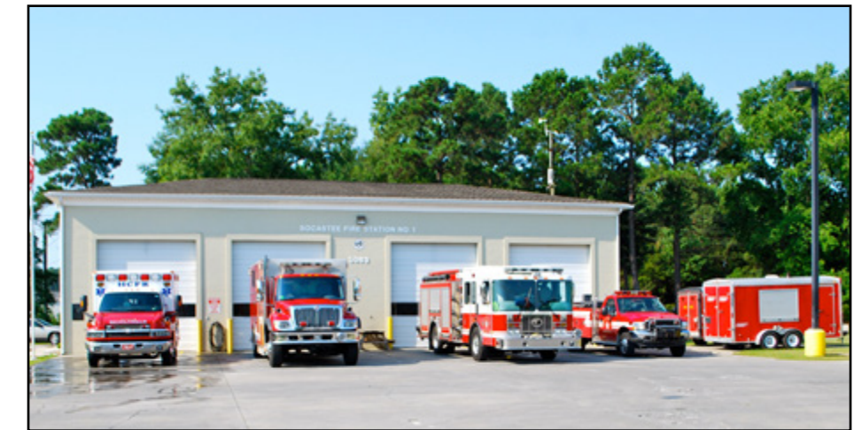
Horry County Fire Socastee Station Source: Horry County Fire and Rescue
