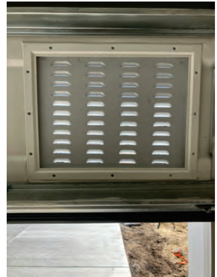
BACK OF NON-ENGINEERED FLOOD VENT
