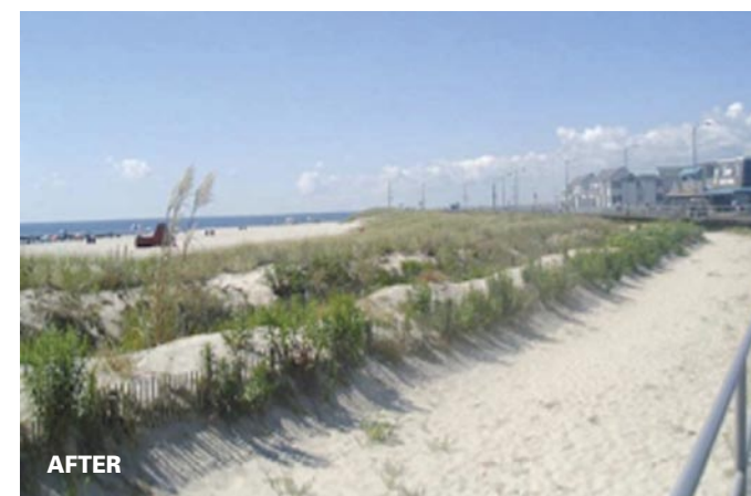
Dunes included in a beach nourishment project act as a protective barrier, preventing flooding and storm damage caused by storm surge, wave runoff, and overtopping. This project was constructed at Ocean City, N.J.
