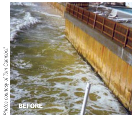
Beach nourishment, which adds sand to the coastal system, protects people and property from the effects of hurricanes and coastal storms by widening a beach and advancing the shoreline seaward. This project was constructed at Panama City Beach, Fla.
