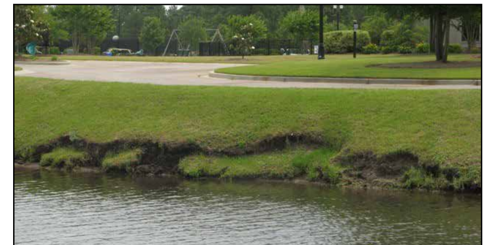
Pond Bank Erosion Photo Credit: Clemson Extension
