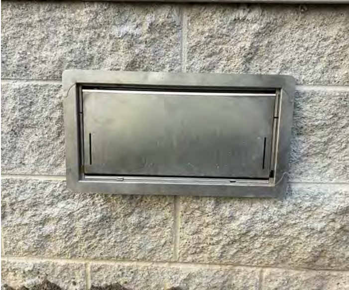
FLOOD VENT IN RIGHT SIDE OF GARAGE
