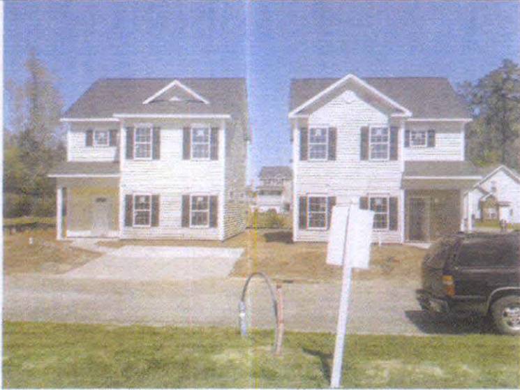
FRONT VIEW (UNIT 20 ON LEFT)
