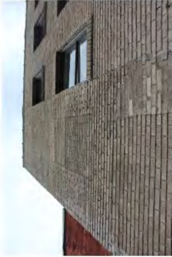
Photo 13 – Scarring in northernmost bay of west elevation
