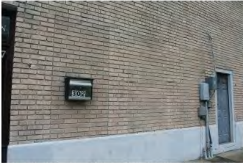
Photo 11 – Scarring between Laurel St. storefront and six-panel door, west elevation looking south
