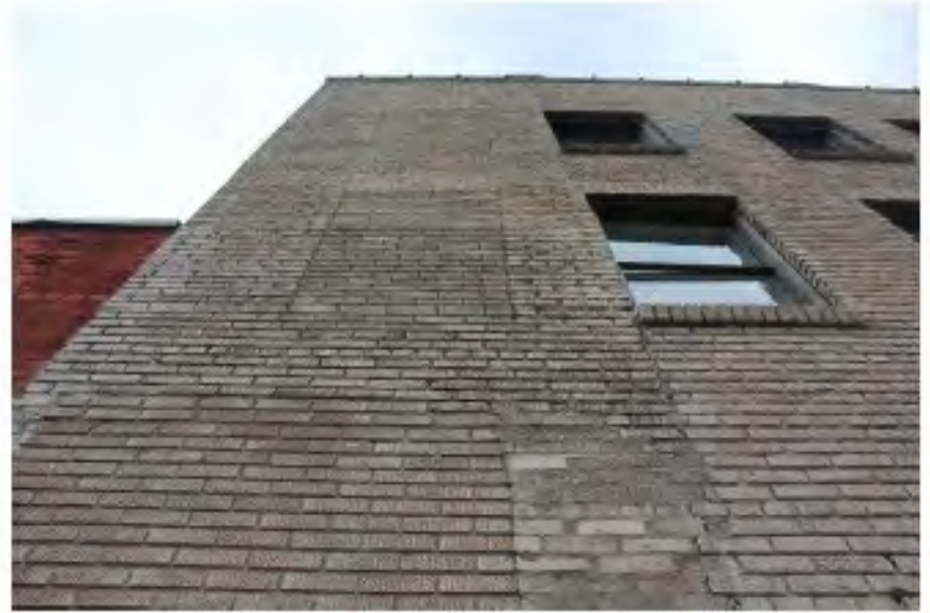
Photo 13 – Scarring in northernmost bay of west elevation
