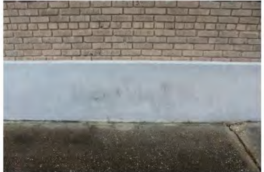
Photo 14 – Stucco water table on west elevation
