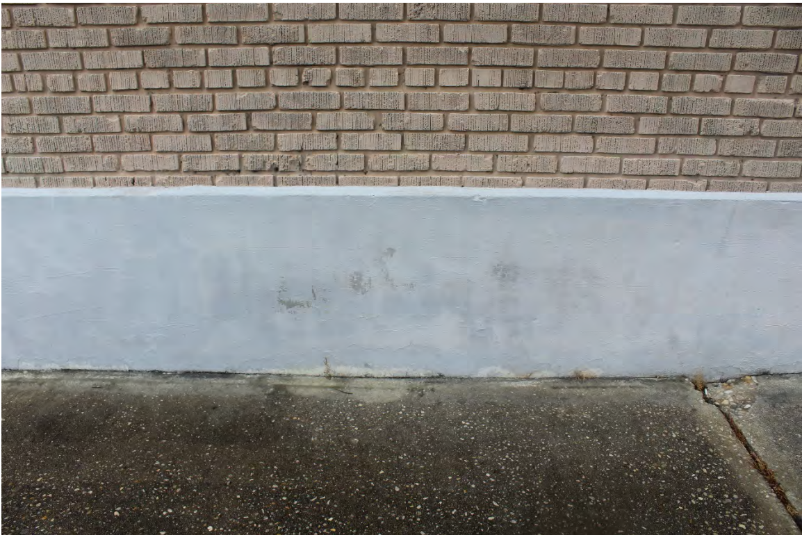
Photo 14 – Stucco water table on west elevation
