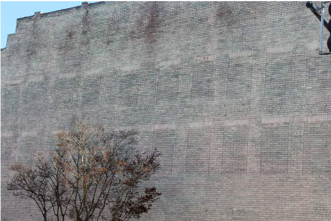
Photo 8 – Window scarring on west elevation
