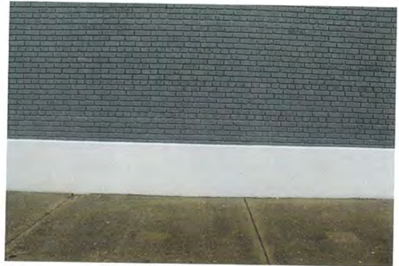
Photo 14 – Stucco water table on west elevation
