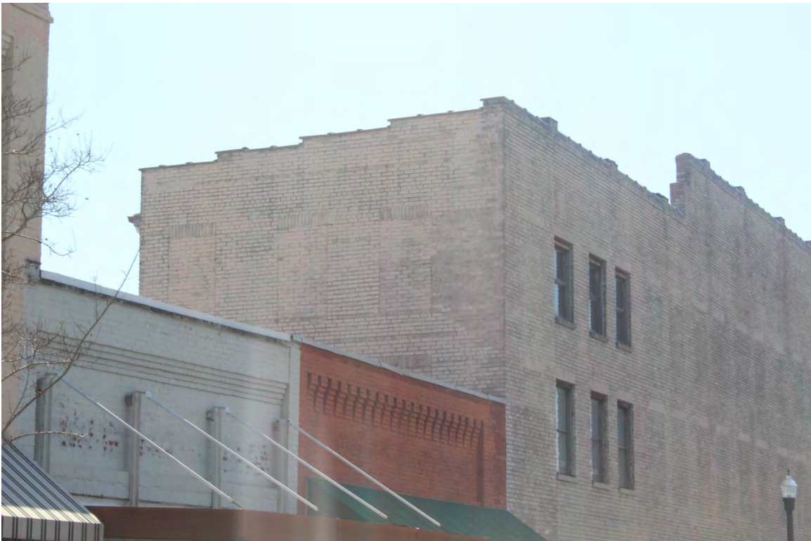
Photo 16 – Window scarring on north elevation
