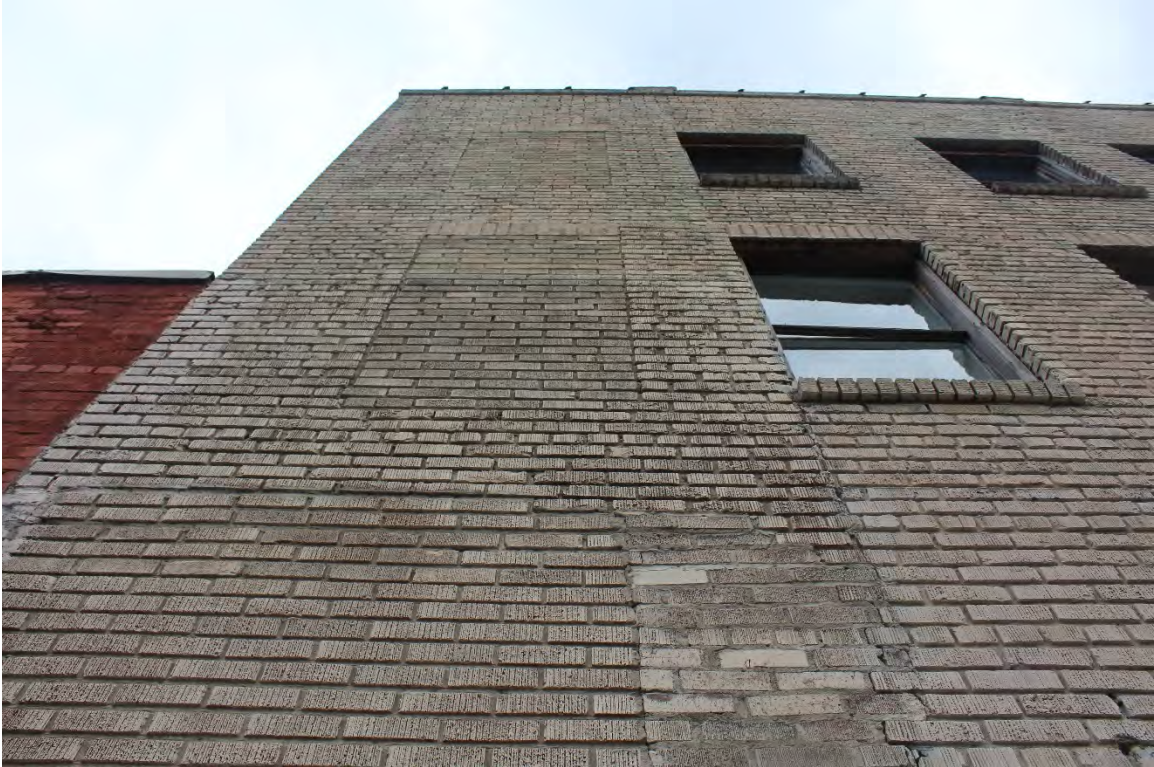
Photo 13 – Scarring in northernmost bay of west elevation
