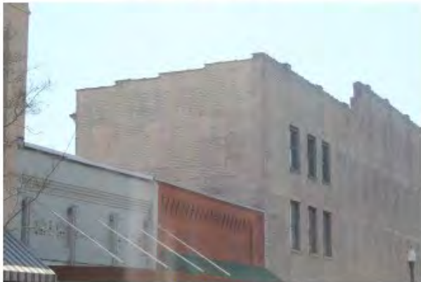
Photo 16 – Window scarring on north elevation
