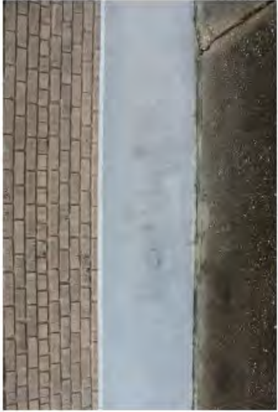
Photo 14 – Stucco water table on west elevation
